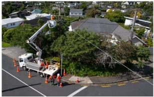
Vector crew cutting down redundant high and low voltage power lines before removing a power pole (Corner of Sylvia Road and Tuhimata Road).
